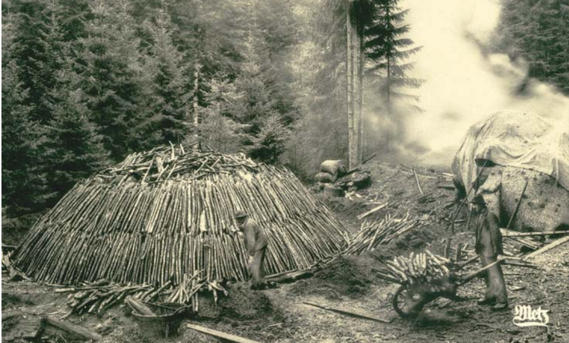
Fig. 13. Wood charcoal production in upright circular kilns. The fuel wood to be charred was arranged upright two to three layers high in hemispherical piles with a diameter of 8 to 12 meters. Background right a burning kiln (Picture: © Metz Publishers, Tübingen/Germany 1905).
